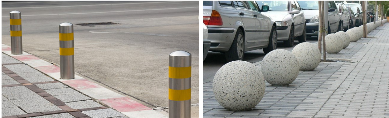
Figure 148. Example of bollards to avoid illegal parking
