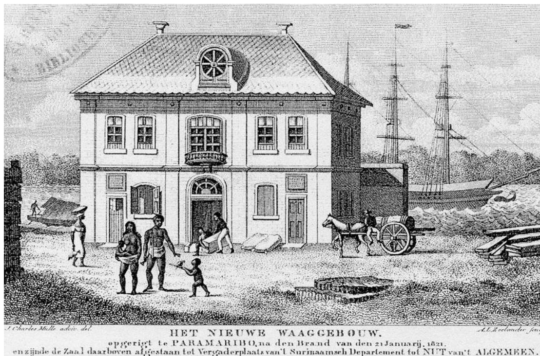
Fig... The Weighing House (Waag) at the Waterfront
