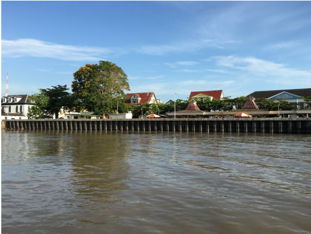
Figure 4-35: Existing Barriers along the Left Bank of Suriname River
