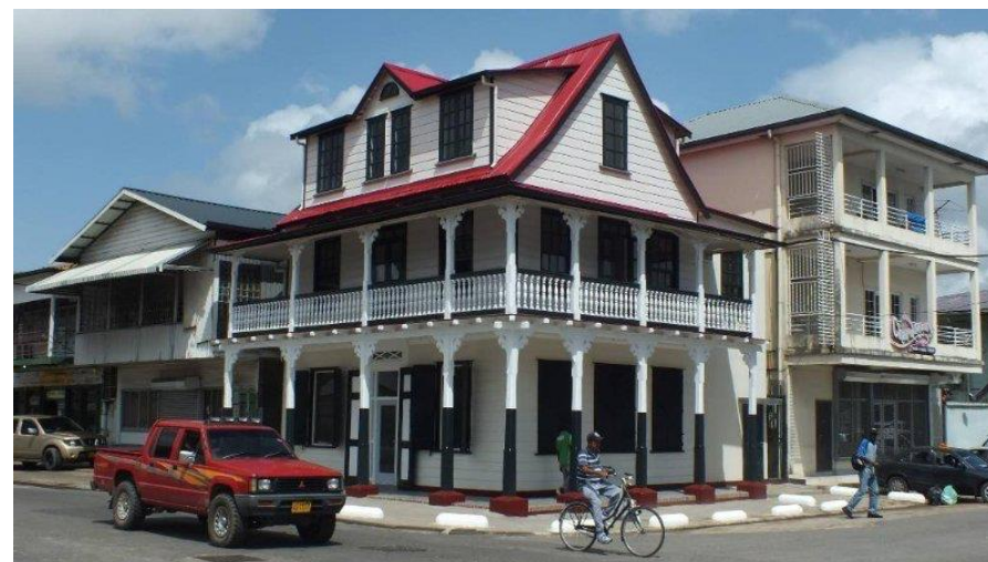
Figure 32: Historic photograph above compared with after 2015 restoration at 116 Zwarthovenbrugstraat below (Maud Houterman, 2019)
